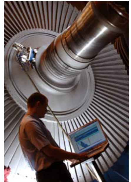
Rotor inspection using state-of-the-art technology by Alstom Inspections Robotics.
